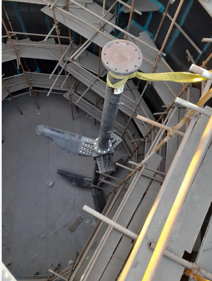
Iron Ore Tailing Agitator, 90kw, 3.7m dia
